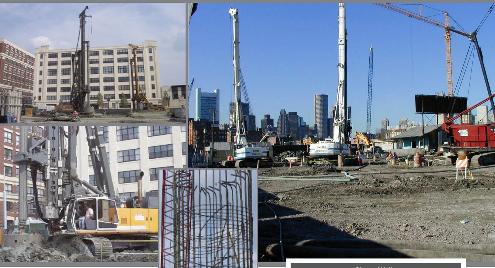
the horizontal reinforcement and span through the diameter of the casing. Once the lower cage is set and secure, the larger diameter cage was lowered over the smaller diameter cage and spliced to the lower section using a combination of Z-bars, lap splices and clips. The spliced cage was then lowered to the design elevation and set on the casing or frame. The cage was suspended on angle iron or
